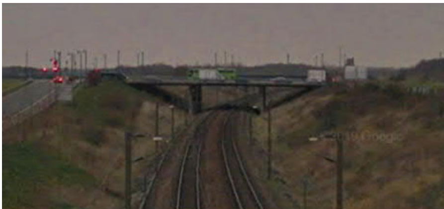
Figur 9 – Bro E10140 Center Boulevard, facade set mod vest.
